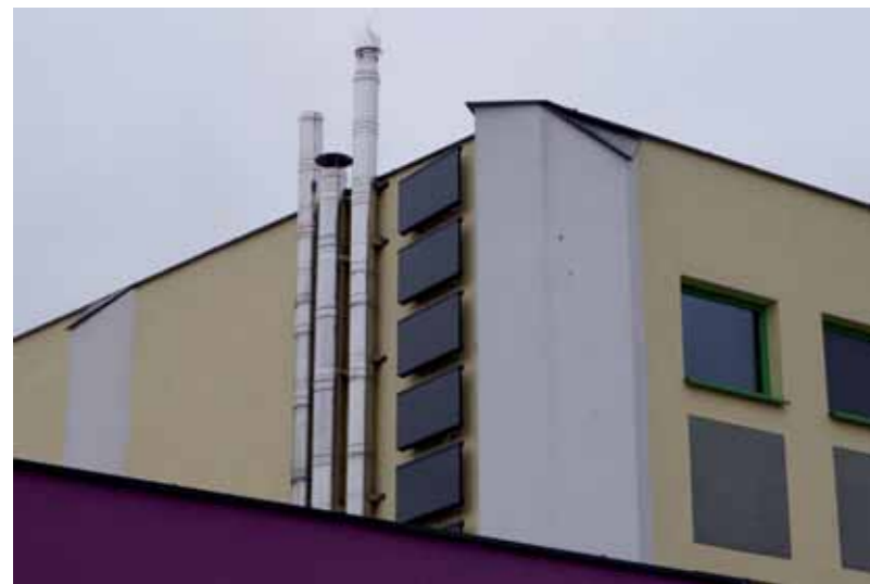
Façade at Sto-ispo (Warsaw) - east-facing
