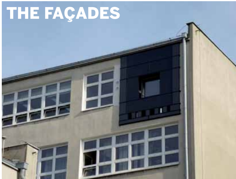
Façade at Lodz University of Technology - west-facing
