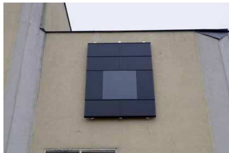
Façade at Sto-ispo (Warsaw) - south-facing
